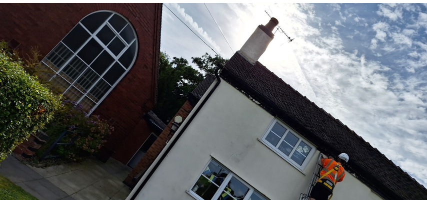
Broadband is finally installed
