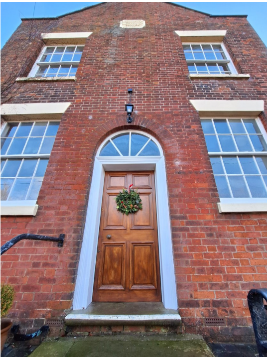
Our newly-varnished chapel door
