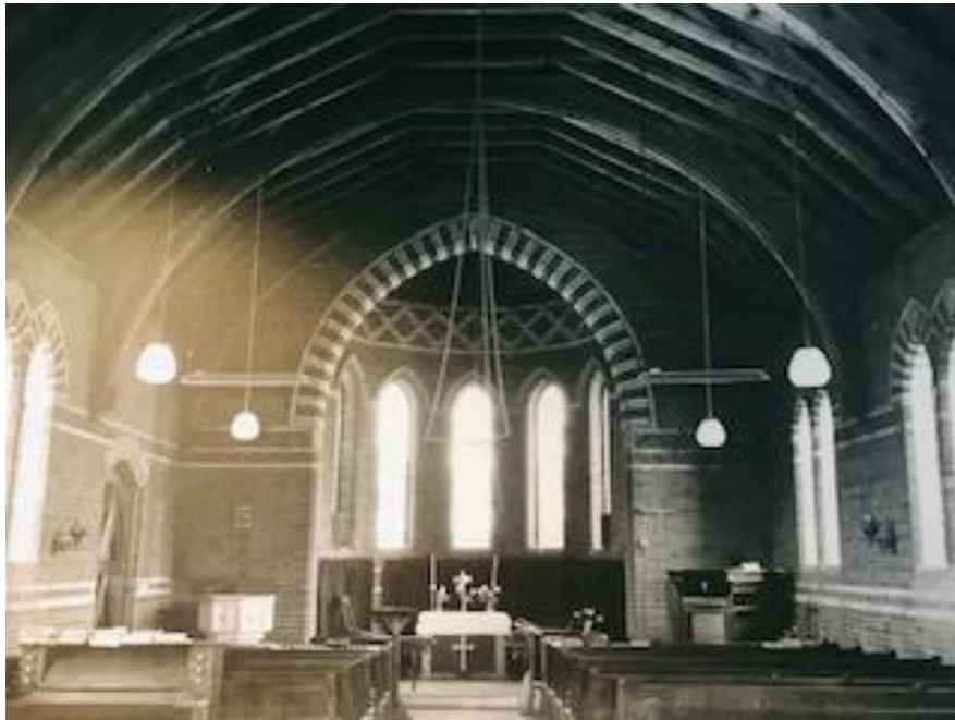
Gressenhall Workhouse chapel
