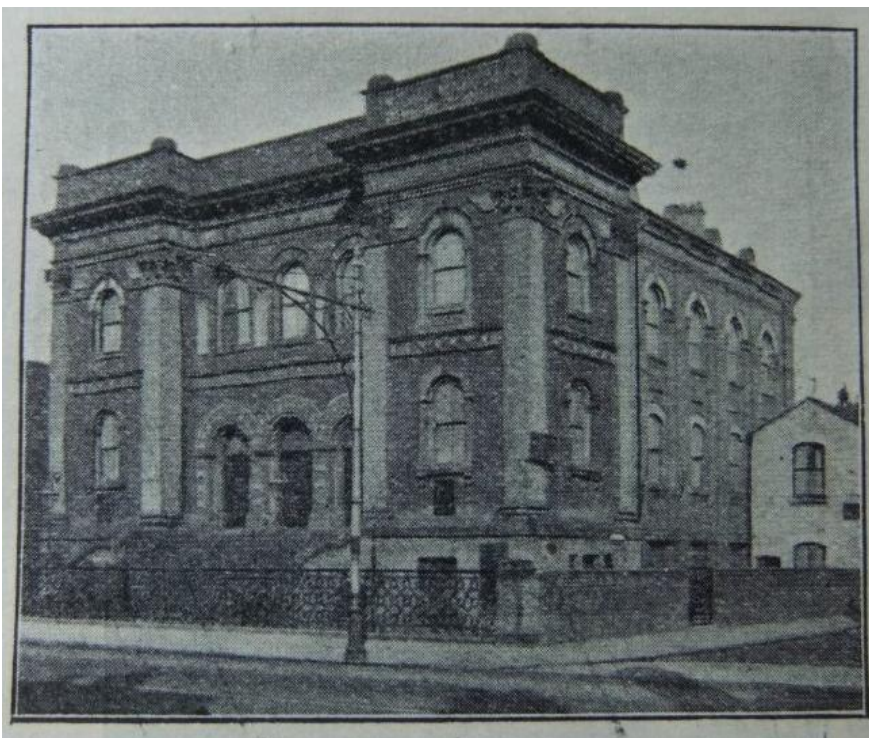
Bright Street chapel, Holderness Road, Hull
